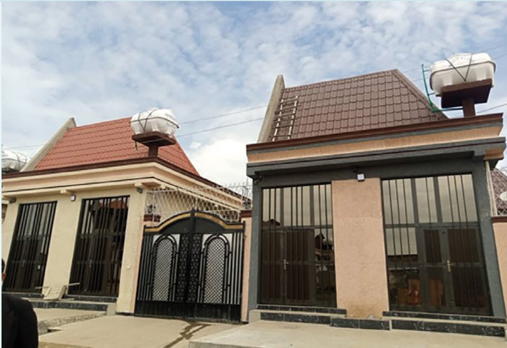
Figure 6: Overhead water storage tanks at a well-off house in Tsedicha kebele (urban) of Dukem town, Ethiopia.
