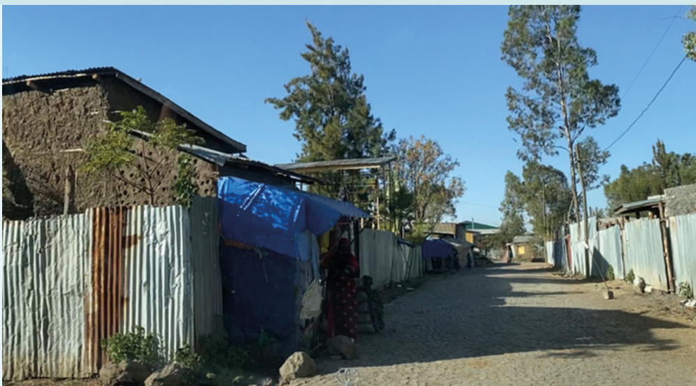
Figure 7: Illegally constructed housing with no land registration certificate results in limited connectivity to the water system, Koticha peri-urban kebele, Dukem town, Ethiopia.
