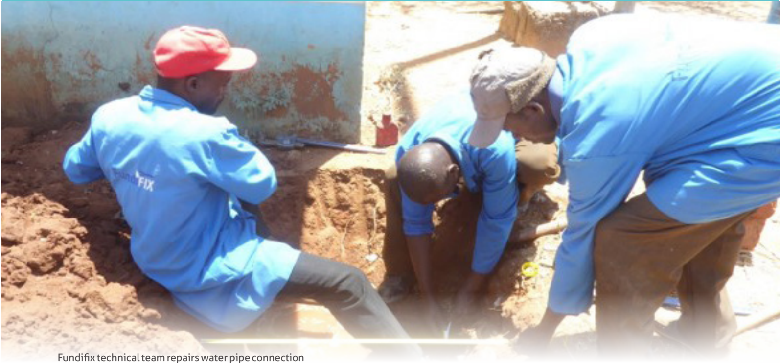
Fundifix technical team repairs water pipe connection
