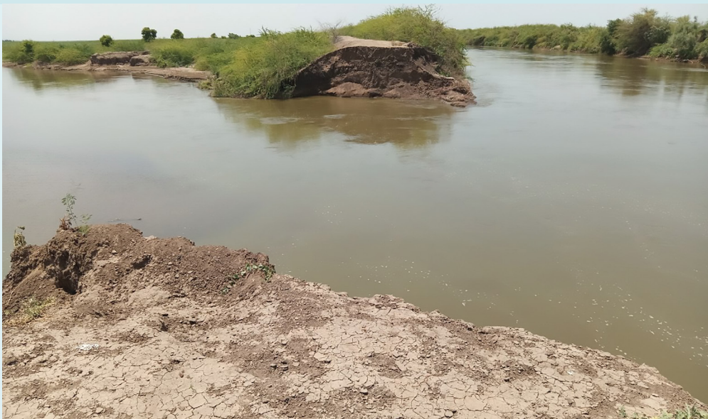
Figure 15: Road washed away in Dubti town due to the 2020 floods, which resulted in abandoning of irrigated land.
