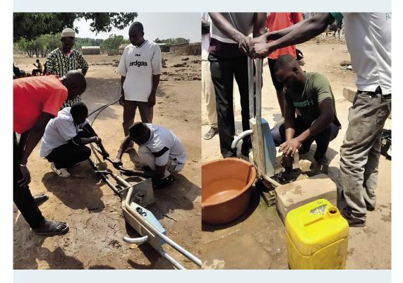
Photos show water service providers repairing handpumps.
