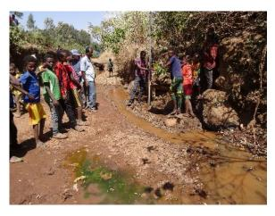
(e) Preparing the bedrock by chipping away the weathered surface and cleaning.
