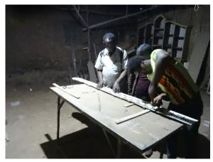
(c) Bolting the wooden planks to the angle iron on the riverbank.
