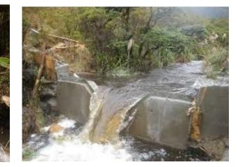
FIGURE 11. (a) A rectangular weir in Kimakia watershed, Kenya. (b) A v-notch weir in Peru. Photos from: Alemseged Tamiru Haile and Buytaert et al. (2014).
