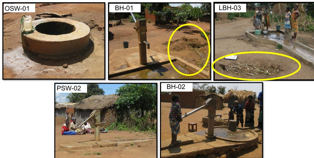
**Fig. 2.** Drinking water sources sampled for this study: Top left: OSW-01 (open shallow well – location 01); centre: HPB-01 (borehole – location 01) with modifications to cement apron highlighted; right: HPB – 03 (borehole near abandoned latrine – location 03) with abandoned latrine pit highlighted; bottom left: HPSW-02 (hand pumped shallow well – location 02); right: HPB-02 (borehole – location 02).
