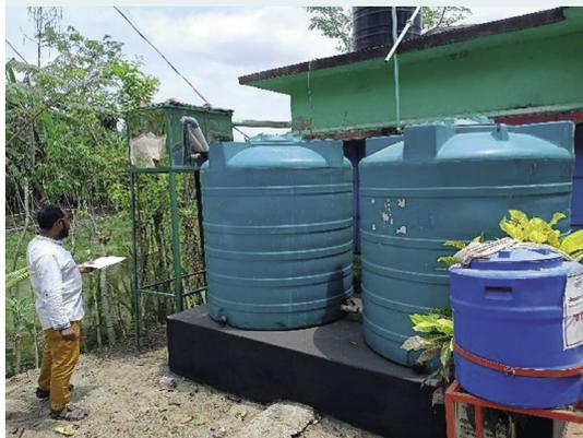
**Passive chlorination.** An in-line chlorination system installed by EOS International in Honduras
