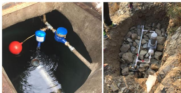
**Figure 1.** (Left) Aquatabs Flo technology installed at the inlet to a reservoir tank. Pretreatment samples were collected from the unchlorinated bypass. (Right) PurAll 100 technology installed in-line just upstream of a reservoir tank. Pretreatment samples were collected from a sampling tap, visible just upstream of the device.
